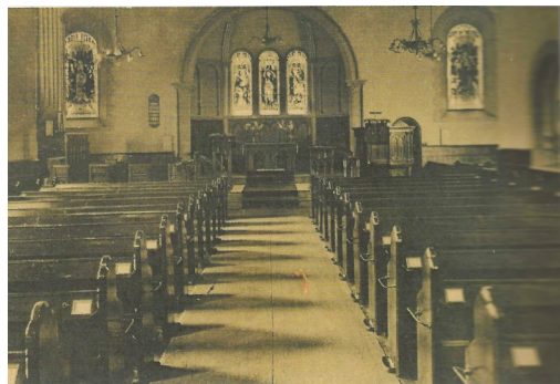
Reigate Congregational Church - demolished in 1972
